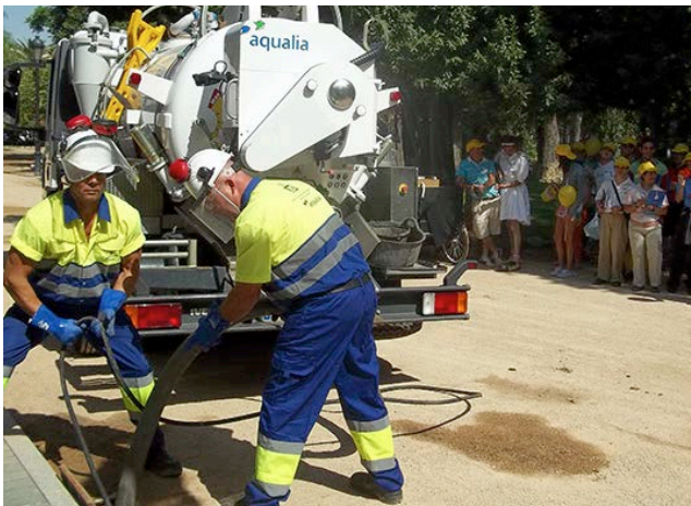
A moment during the demonstration of how manholes are cleaned.
